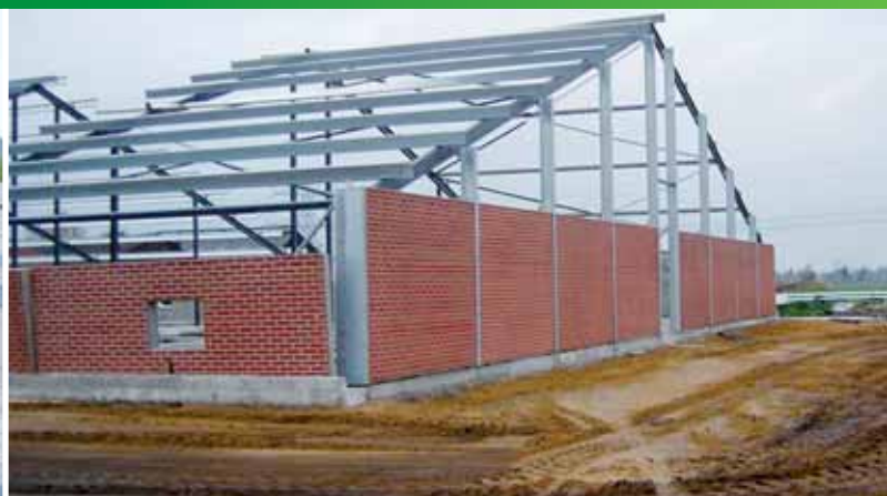
Steel purlins enable a greater span. The precast elements have a very high insulation value and enable pig houses to be constructed in a very short time.
