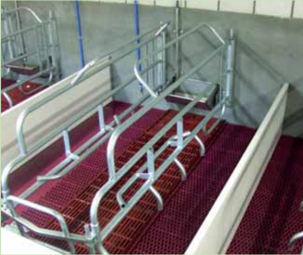
The combination of slatted floors with a soft coating for the piglets and cast iron grates under the sow is the best farrowing pen floor system.
