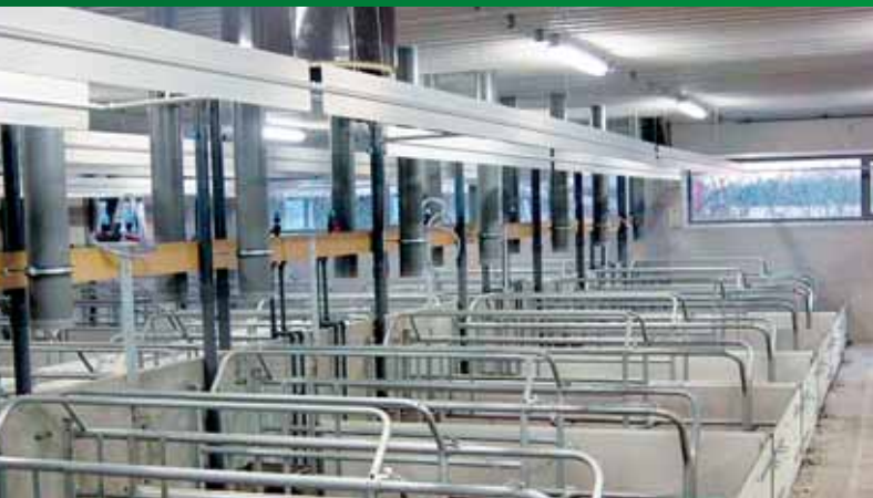
A "Soft-Air" ventilation ceiling with twin pipe heating pipes and a "cool nose" system, for an ideal climate year round!
